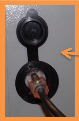
Standard 110V Power Receptacle
